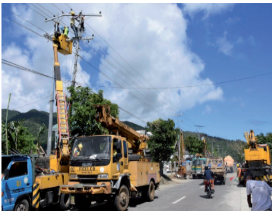
Line rehabilitation and power restoration works being done in the Province of Catanduanes
